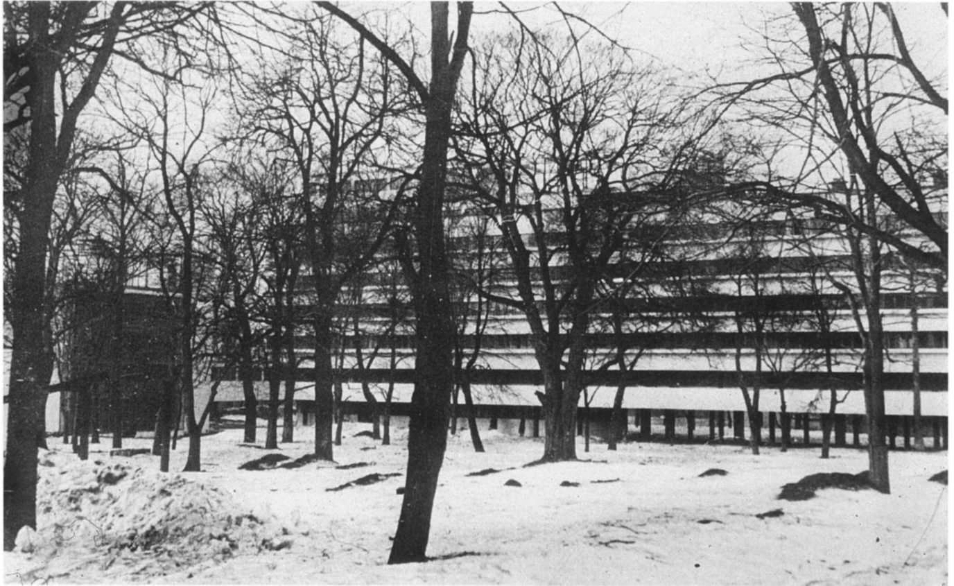
FIGURE 11: Winter view of the Narkomfin Communal House, early 1930s
