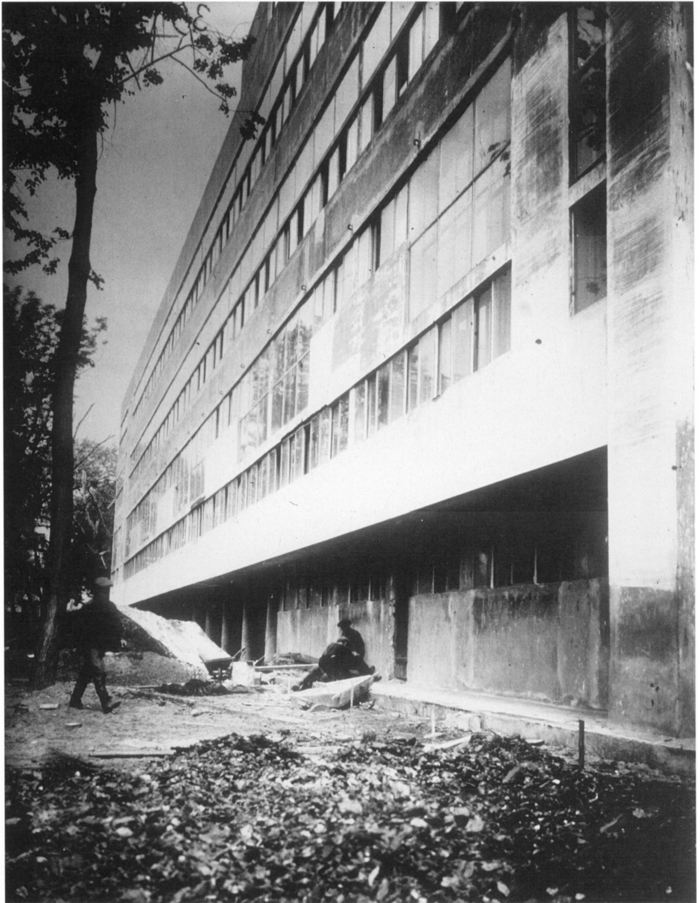
FIGURE 3: View of the west facade during construction, 1929
