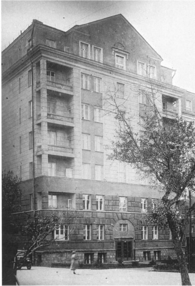
FIGURE 14: Second-phase House of the Council of People's Commissars designed by the Stalinist classicist Leontovich, 1935
